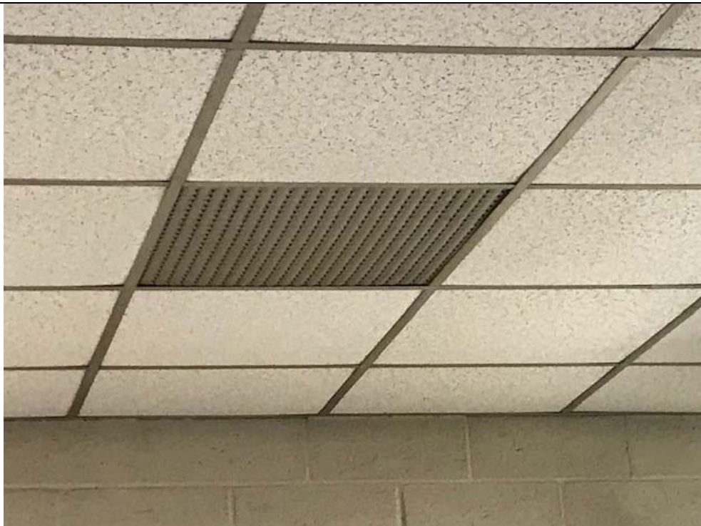
Photo 2: Library – Ceiling mounted air grills clean and free of dust.
