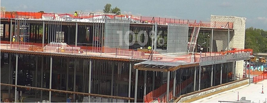
Exterior Framing South
