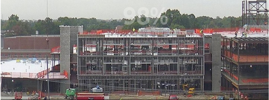
Exterior Framing North
