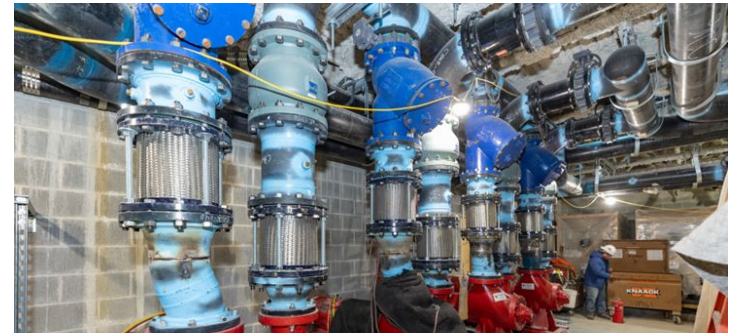
Mechanical Equipment Installation
