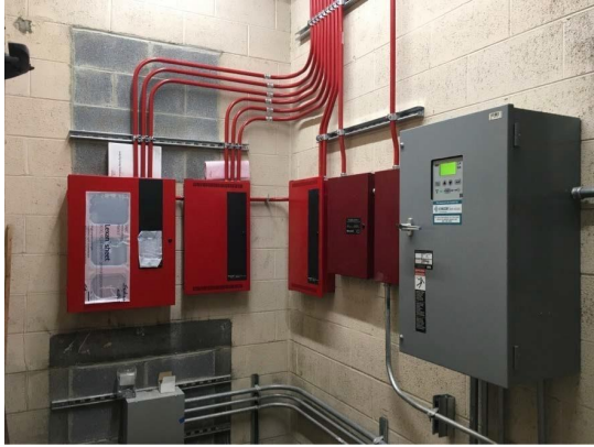
Digital, Addressable Fire Detection Panels
