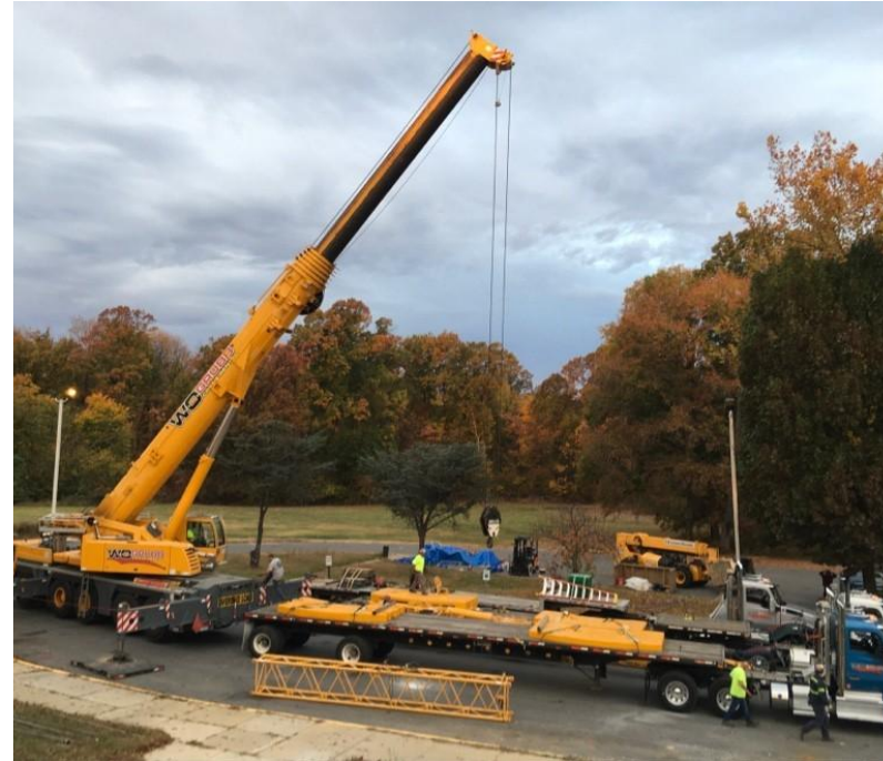
Delivery of HVAC Units
