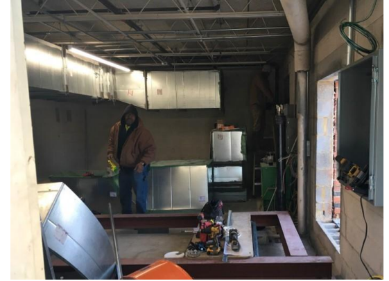
Structural Steel Framing for Penthouse Equipment
