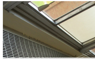
Typical Existing Hot Water Radiator
