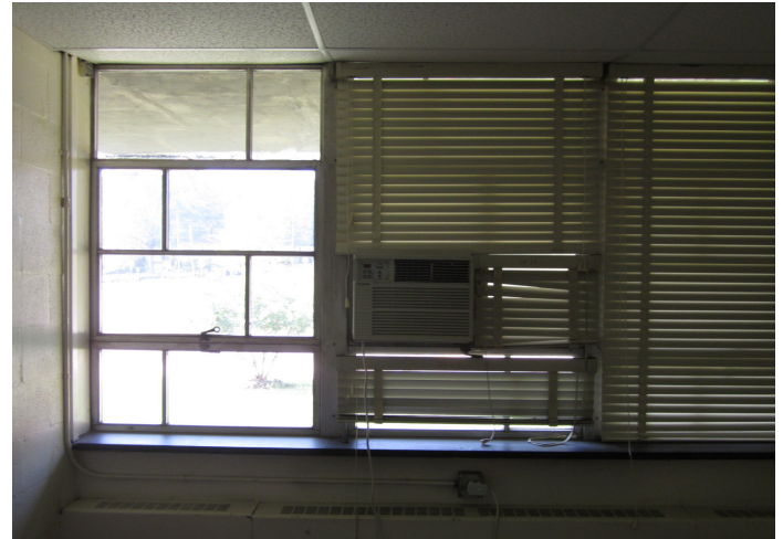
Cloudy lexan windows, venetian blinds and window mounted AC unit (typical).
