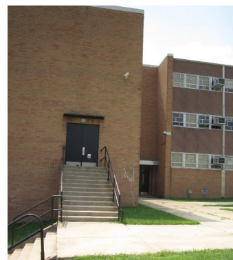
Exterior exit stair at gym.
