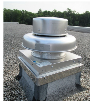
Roof Mounted Exhaust Fan
