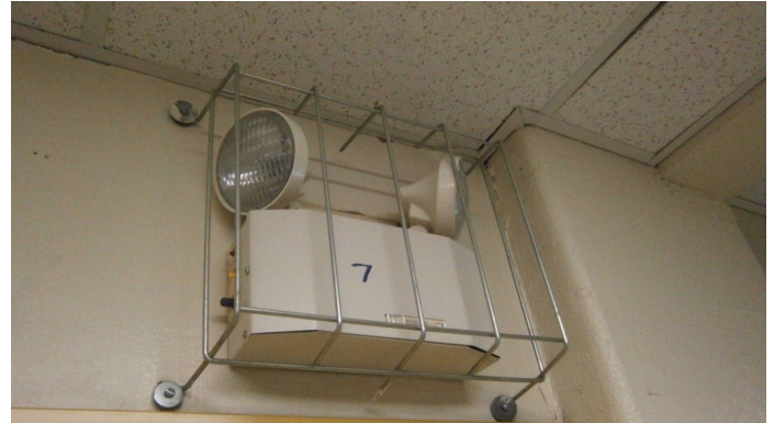
Typical Emergency battery pack unit
