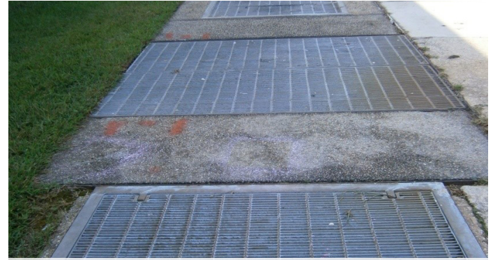
Underground Vault containing PEPCO Step-Down Transformer
