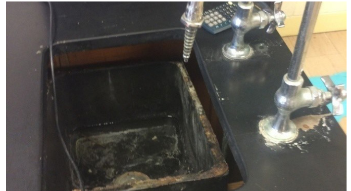
Broken Lab Sink Basin
