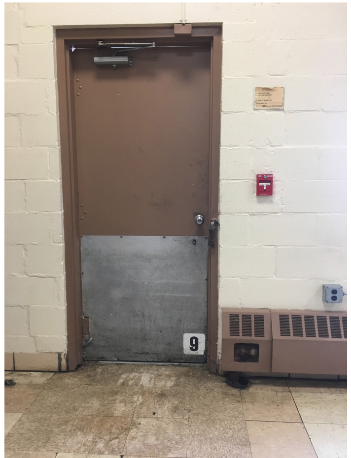
Exterior door in cafeteria
