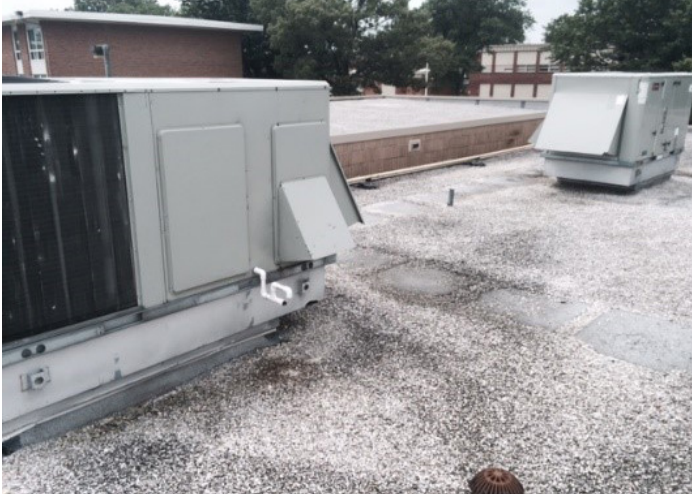
Rooftop units in good condition
