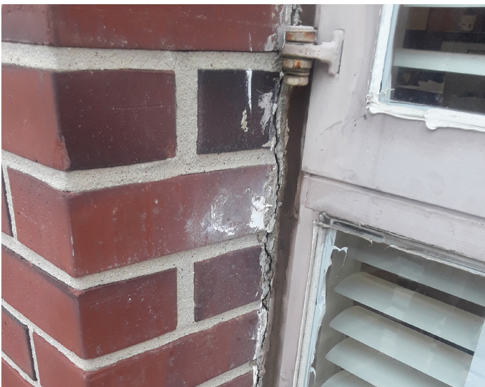
Sealant deteriorating at windows
