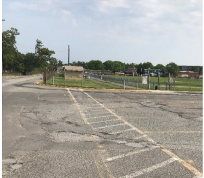
Damaged asphalt
