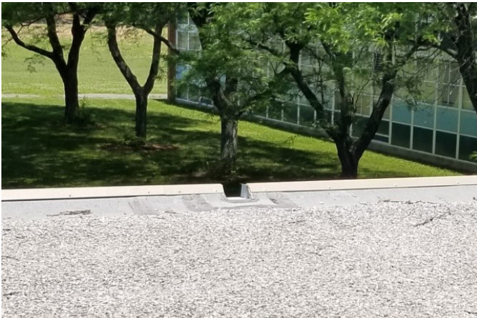
Scuppers at roof edge
