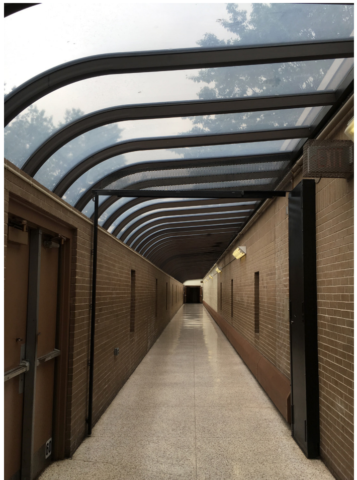
Walkway between high school and CTE
