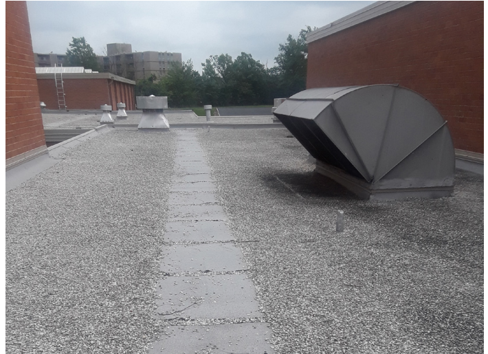
Walkway on roof
