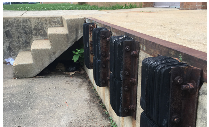
Bumpers at loading dock
