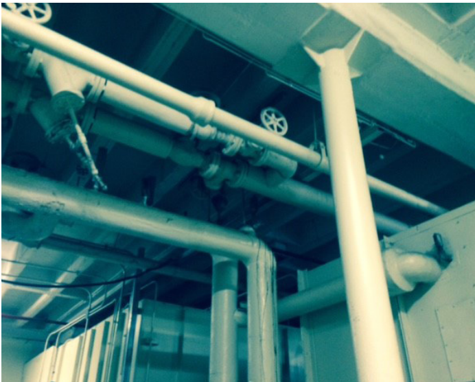
Typical Built up AHU on 1st and 2nd floor
