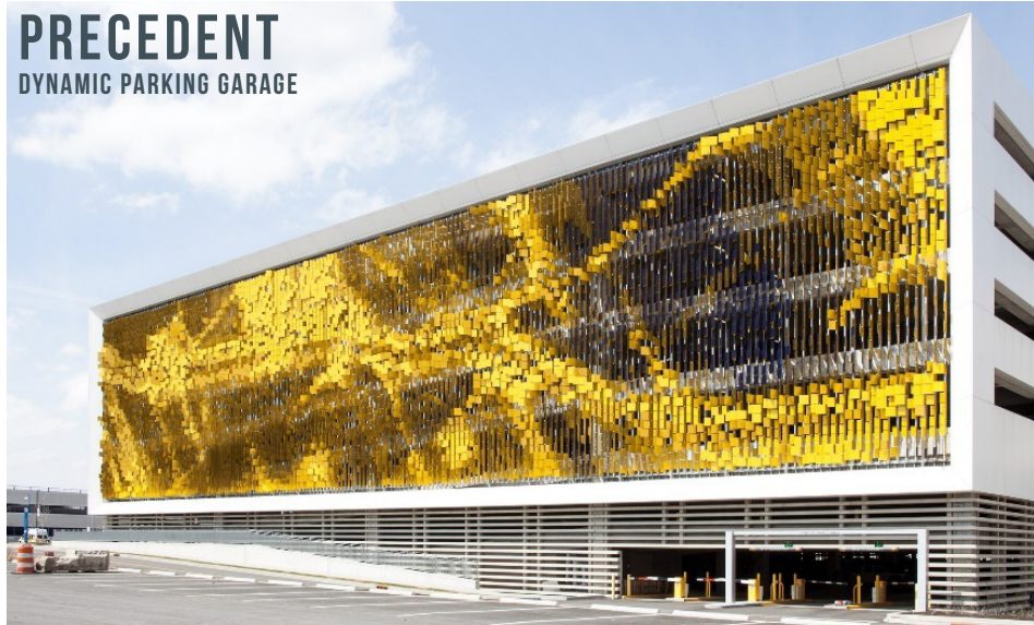
ESKENAZI HOSPITAL GARAGE, URBANA STUDIOS
