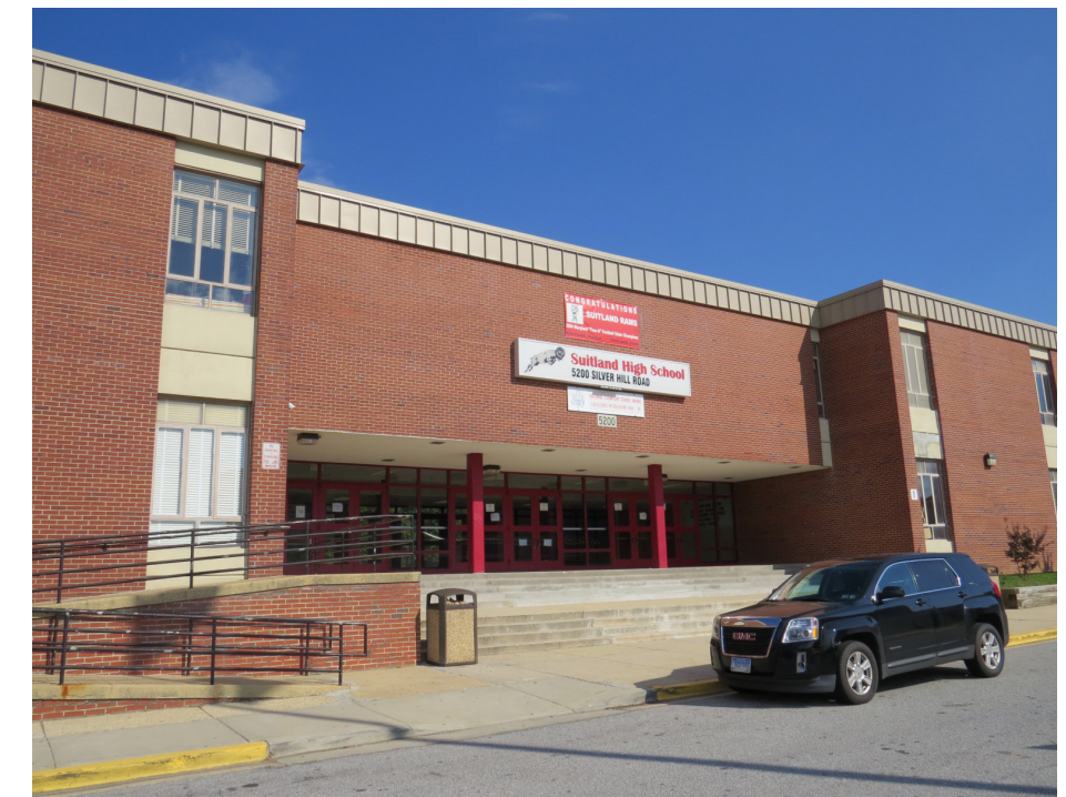
Existing Suitland High School - Main Entrance
