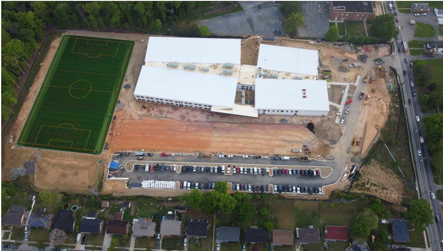
Aerial Site View; Photo Taken Late April
