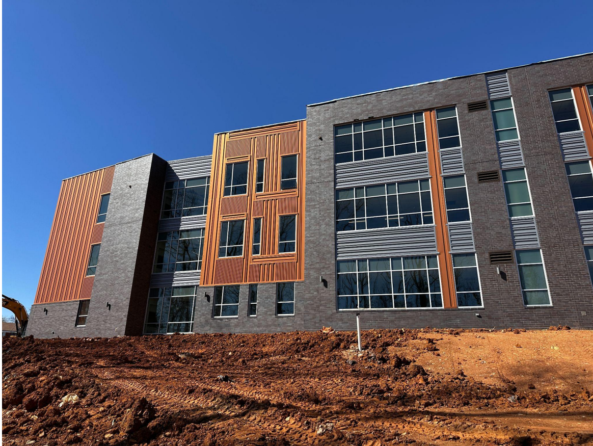
East side of building show 3 story classroom wing
