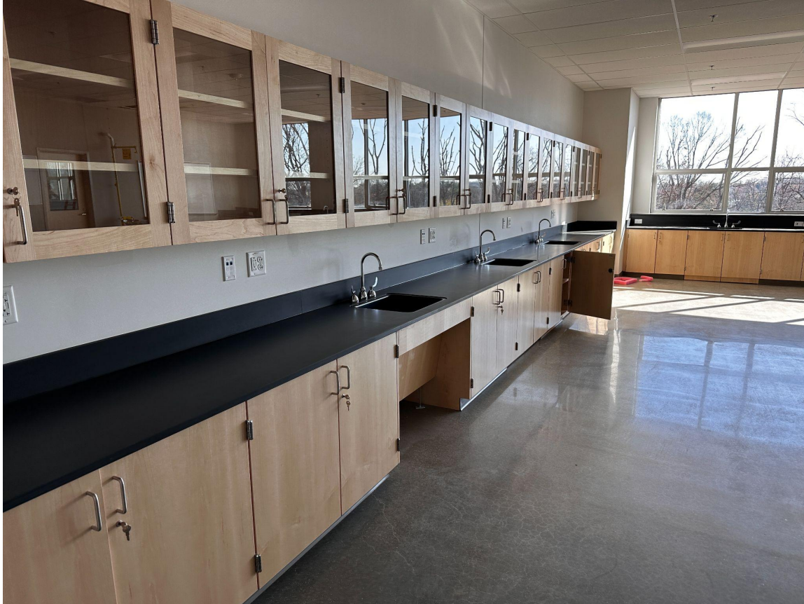
Casework installed in science classroom
