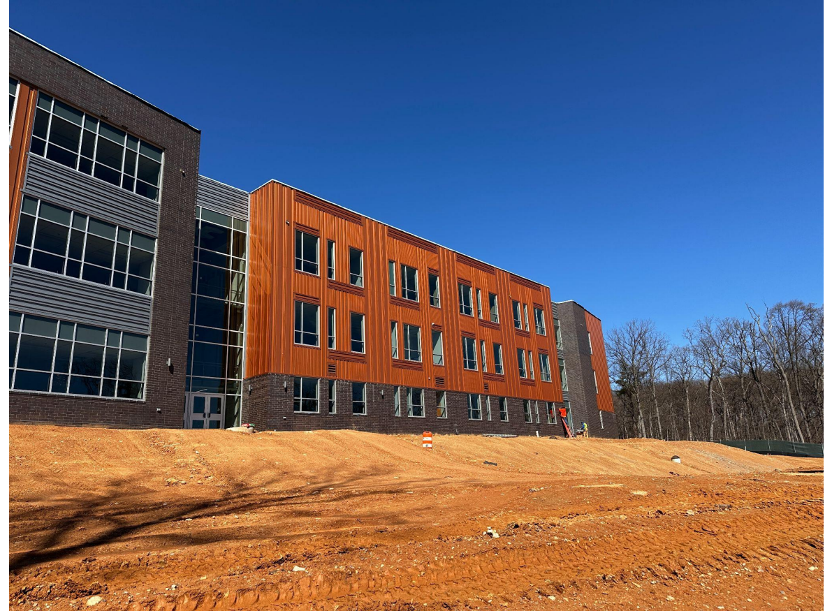
Continuation of 3 classroom building wing
