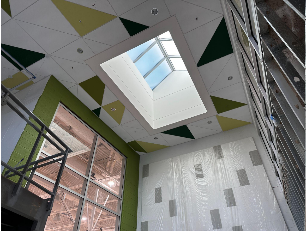
Entry Space Skylight & Ceiling
