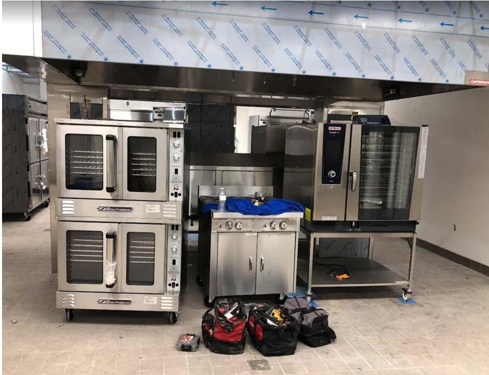
Kitchen Equipment Install
