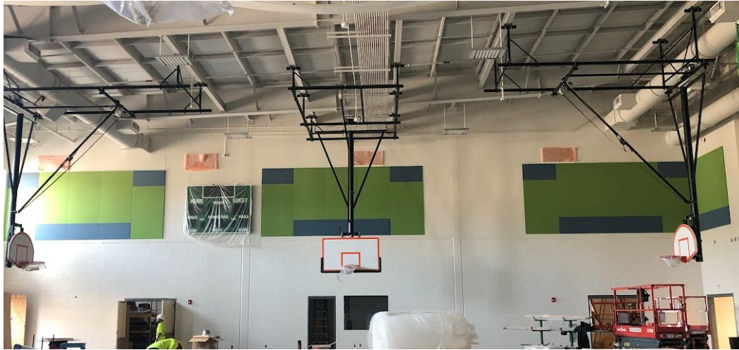
Gymnasium Basketball Hoop Install
