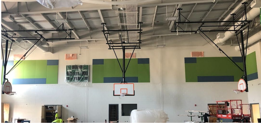
Gymnasium Basketball Hoop Install
