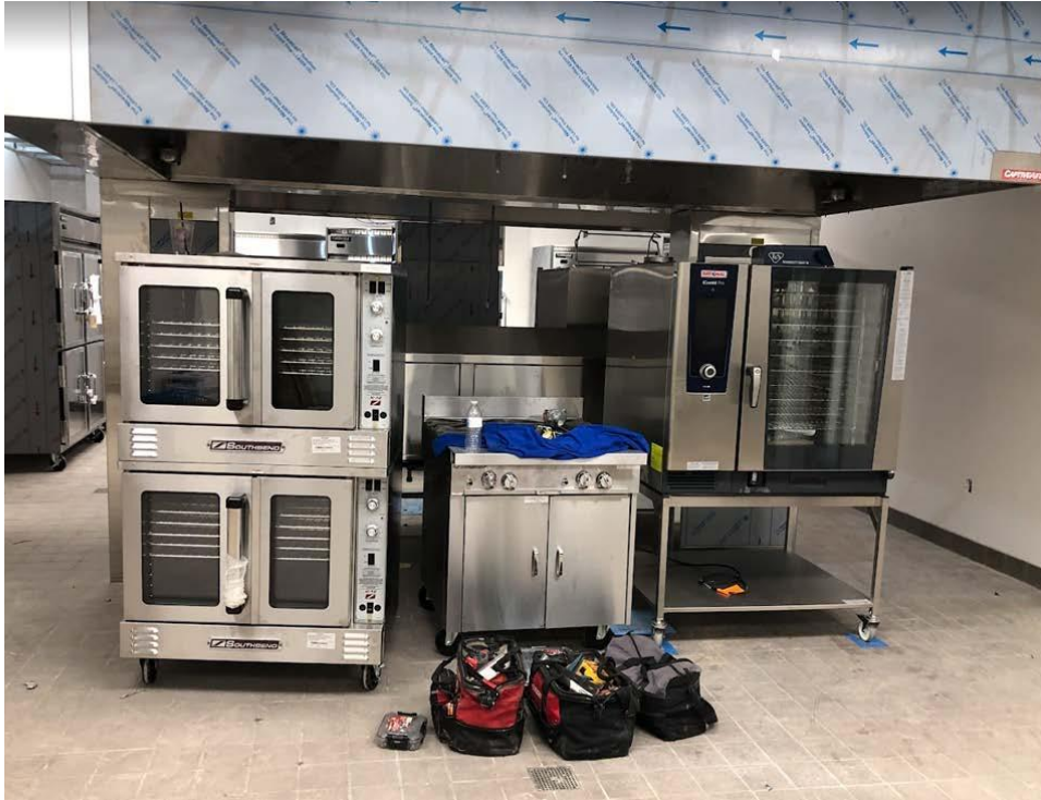
Kitchen Equipment Install
