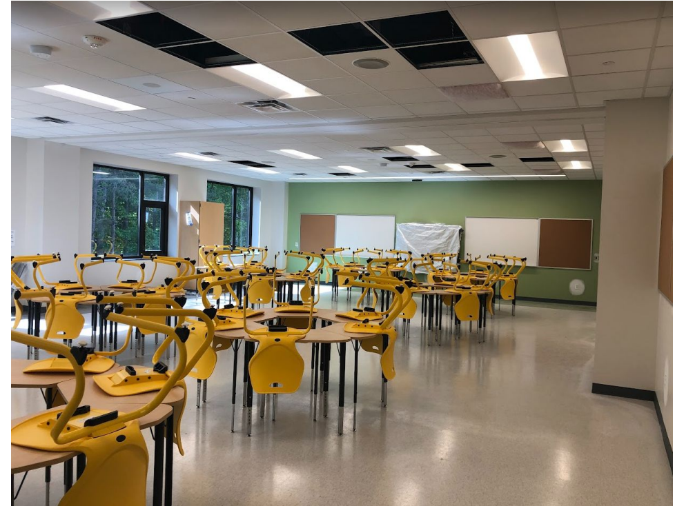
Typical Classroom / FF&E Install
