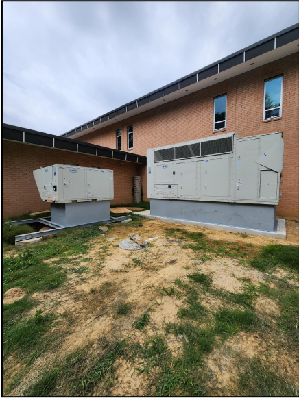
Picture Captions From Left to Right: Newly installed mechanical equipment on new concrete pads, newly installed VAV Boxes, Newly installed mechanical equipment on new concrete pads and steel dunnage, and images of convectors and various materials stored in gymnasium.
