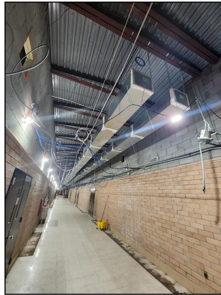
Picture Captions From Left to Right: New AHU installed on new concrete pad, new sprinkler line rough-in and mechanical rough-ins through corridors, newly installed ductwork and trunklines, and rigging image of newly installed mechanical equipment.
