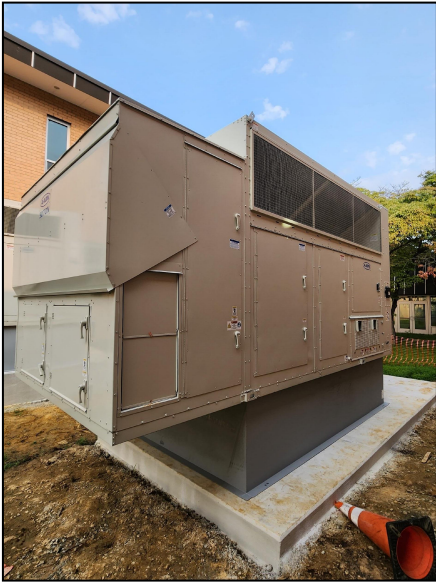
Picture Captions From Left to Right: New AHU installed on new concrete pad, new sprinkler line rough-in and mechanical rough-ins through corridors, newly installed ductwork and trunklines, and rigging image of newly installed mechanical equipment.
