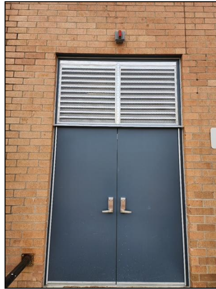
Picture Captions From Left to Right: Images of New Exterior Metal Doors and Frames Installation at Various Locations around James Madison Middle. Image 4 contains a new louver installed above the new door and frame.
