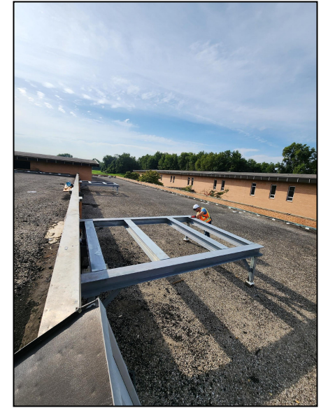
Picture Captions From Left to Right: Newly installed mechanical equipment on new concrete pads and images of new roof steel dunnages for RTU installation.
