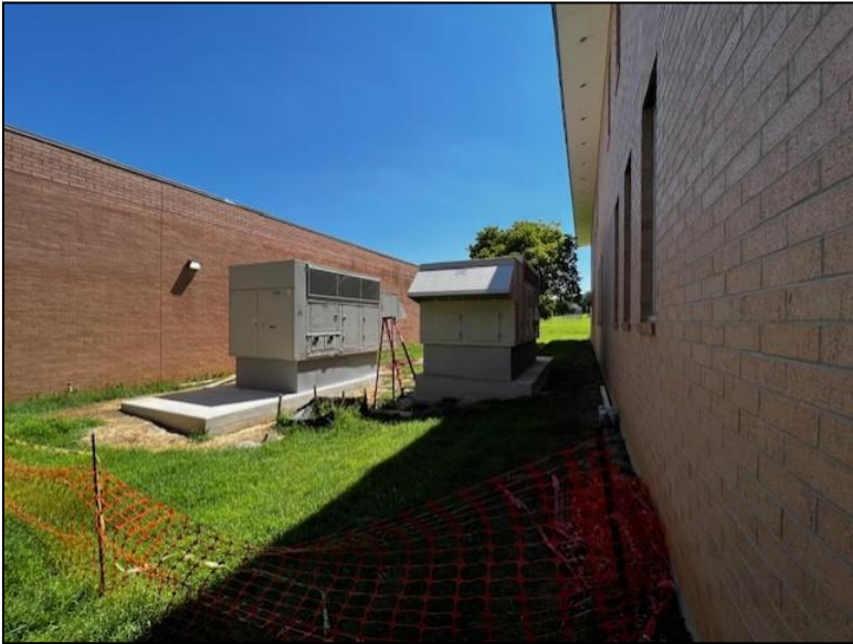
Picture Captions From Left to Right: Newly installed mechanical equipment on new concrete pads and images of new roof steel dunnages for RTU installation.
