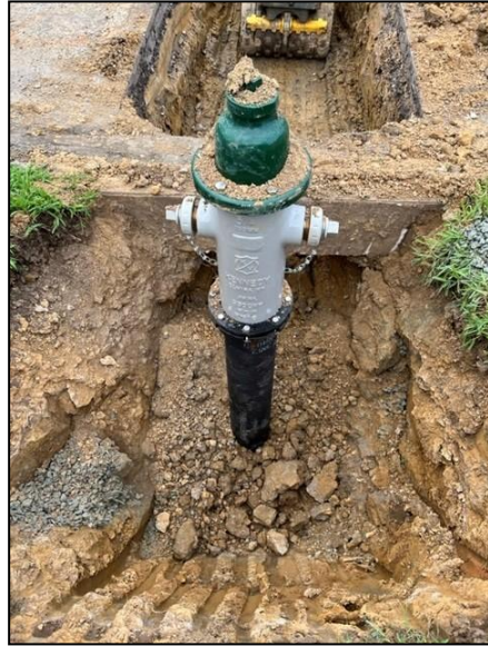
Picture Captions From Left to Right: [Images of the New Water Main addition from Woodyard Road into James Madison Mechanical Room] New 6" Water Main, New Fire Hydrant associated with Water Main, Vault Installation Image, Mechanical Room Fire Pump for Sprinkler System, and Fire Sprinkler Branch Lines for Sprinkler System
