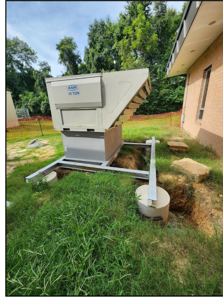
Picture Captions From Left to Right: Newly installed mechanical equipment on new concrete pads, newly installed VAV Boxes, Newly installed mechanical equipment on new concrete pads and steel dunnage, and images of convectors and various materials stored in gymnasium.
