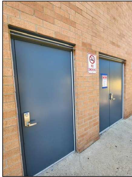
Picture Captions From Left to Right: Images of New Exterior Metal Doors and Frames Installation at Various Locations around James Madison Middle. Image 4 contains a new louver installed above the new door and frame.
