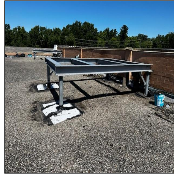
Picture Captions From Left to Right: Newly installed mechanical equipment on new concrete pads and images of new roof steel dunnages for RTU installation.
