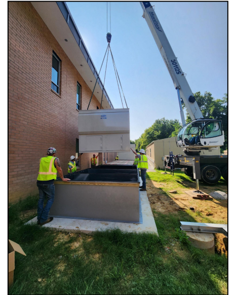
Picture Captions From Left to Right: New AHU installed on new concrete pad, new sprinkler line rough-in and mechanical rough-ins through corridors, newly installed ductwork and trunklines, and rigging image of newly installed mechanical equipment.
