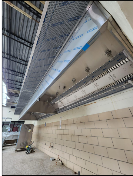
Picture Captions From Left to Right: Newly installed mechanical equipment on new pad, newly installed Kitchen Hood, and mechanical/sprinkler/controls and Low voltage rough-in through various corridors
