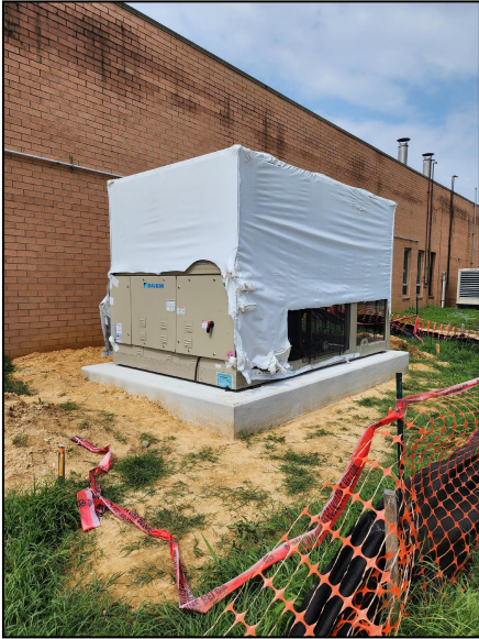
Picture Captions From Left to Right: Newly installed mechanical equipment on new pad, newly installed Kitchen Hood, and mechanical/sprinkler/controls and Low voltage rough-in through various corridors
