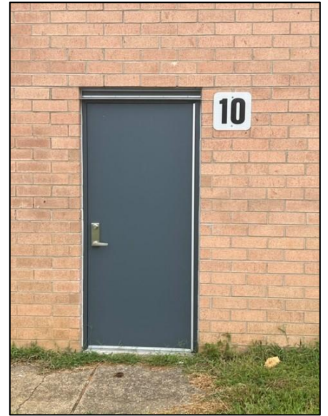
Picture Captions From Left to Right: Images of New Exterior Metal Doors and Frames Installation at Various Locations around James Madison Middle. Image 4 contains a new louver installed above the new door and frame.
