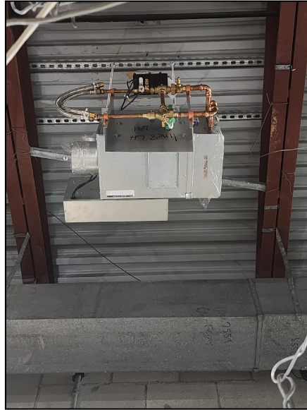
Picture Captions From Left to Right: Newly installed mechanical equipment on new concrete pads, newly installed VAV Boxes, Newly installed mechanical equipment on new concrete pads and steel dunnage, and images of convectors and various materials stored in gymnasium.
