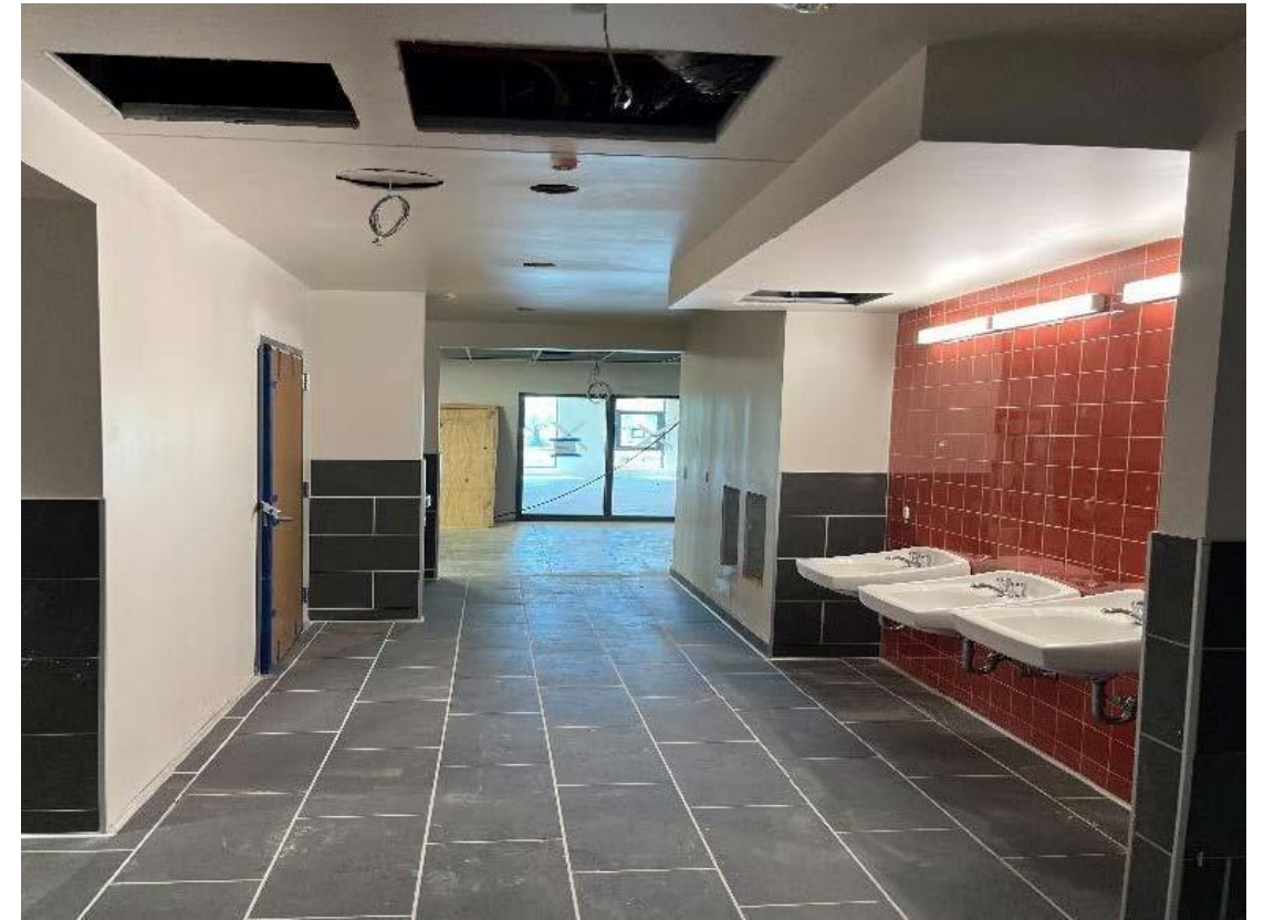
Group Toilet - Ceramic Tile, VCT Install
