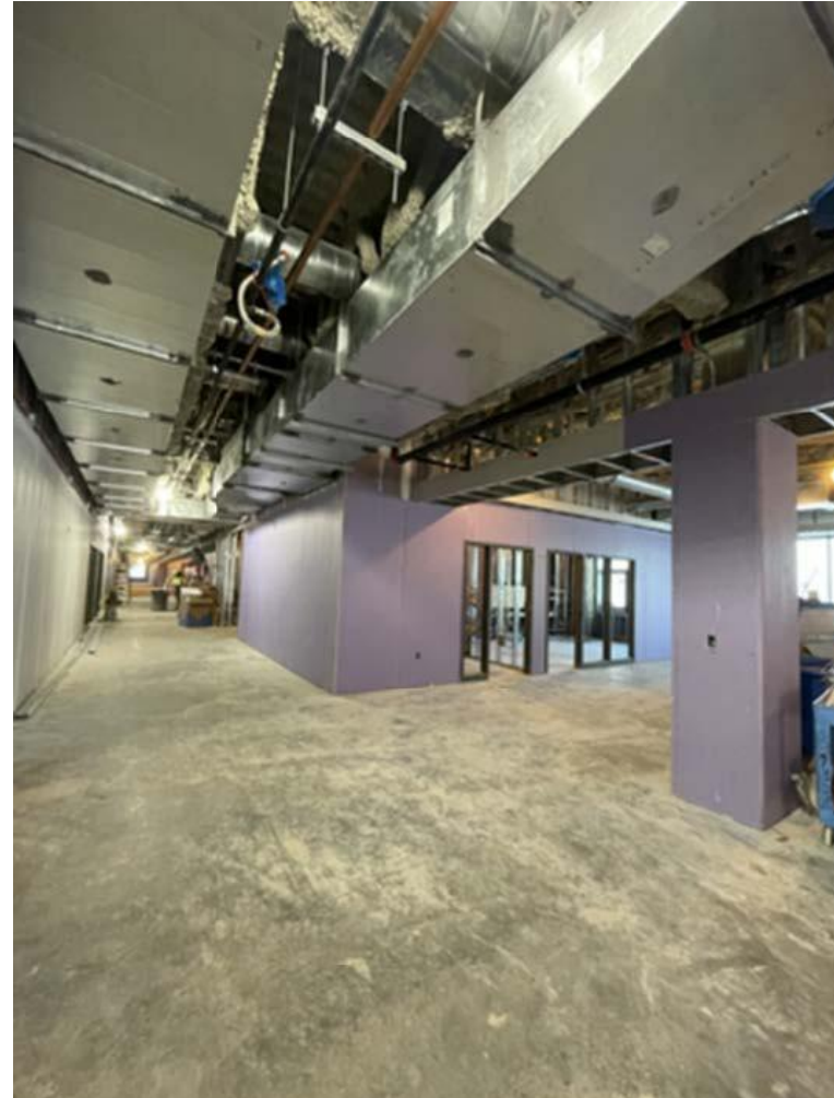
2nd Floor (4-Story Tower).
