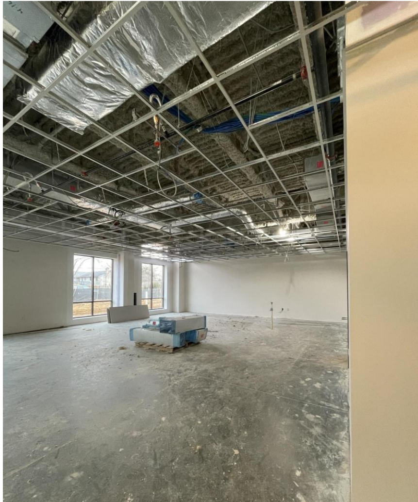
Classroom on level 1 of the north area.
