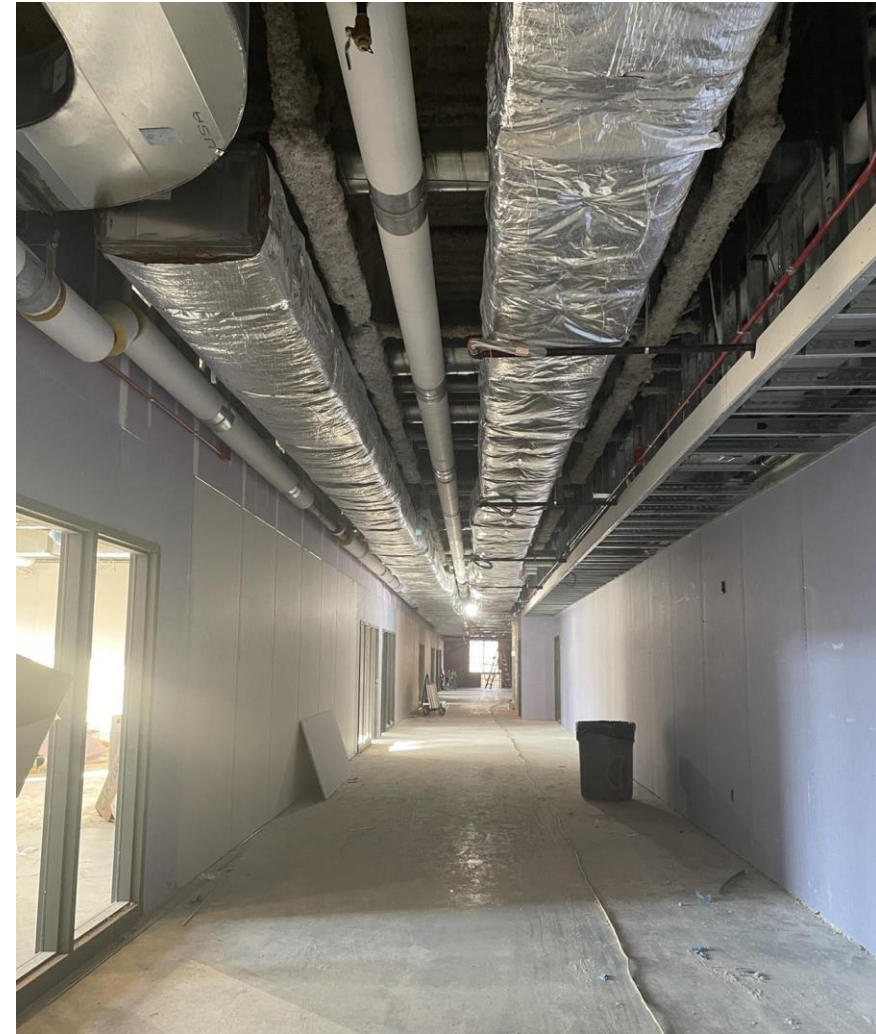
Corridor on level 2 of the 4-story tower.
